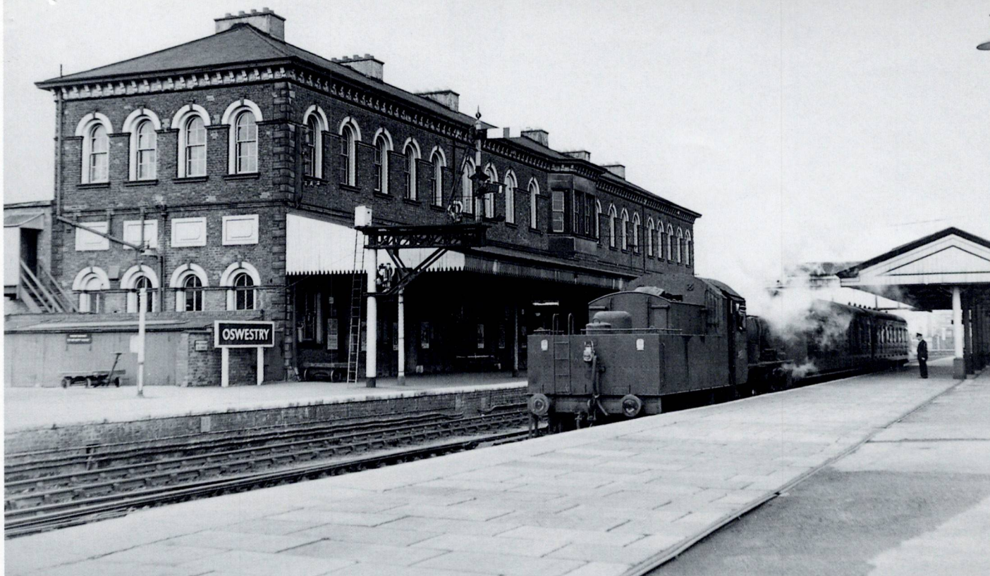
Above: On 27 October 1962 the 2-coach 12.40pm train for Llanfyllin is pictured at Oswestry with Ivatt '2MT' 2-6-0 No 46509 in charge — the regular motive power for these branch trains at this period in time. The scene also provides an excellent view of the substantial two-storey red brick Cambrian station building on the up side of the line at Oswestry with its six squat chimneys, together with the large canopy that protected passengers on the platform from the elements. This building contained a booking office, waiting-rooms, refreshment room, and telegraph office. E. Wilmshurst
