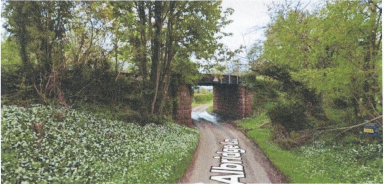
Looking South through the bridge spanning Albridge Lane. [Google Streetview, April 2024]
