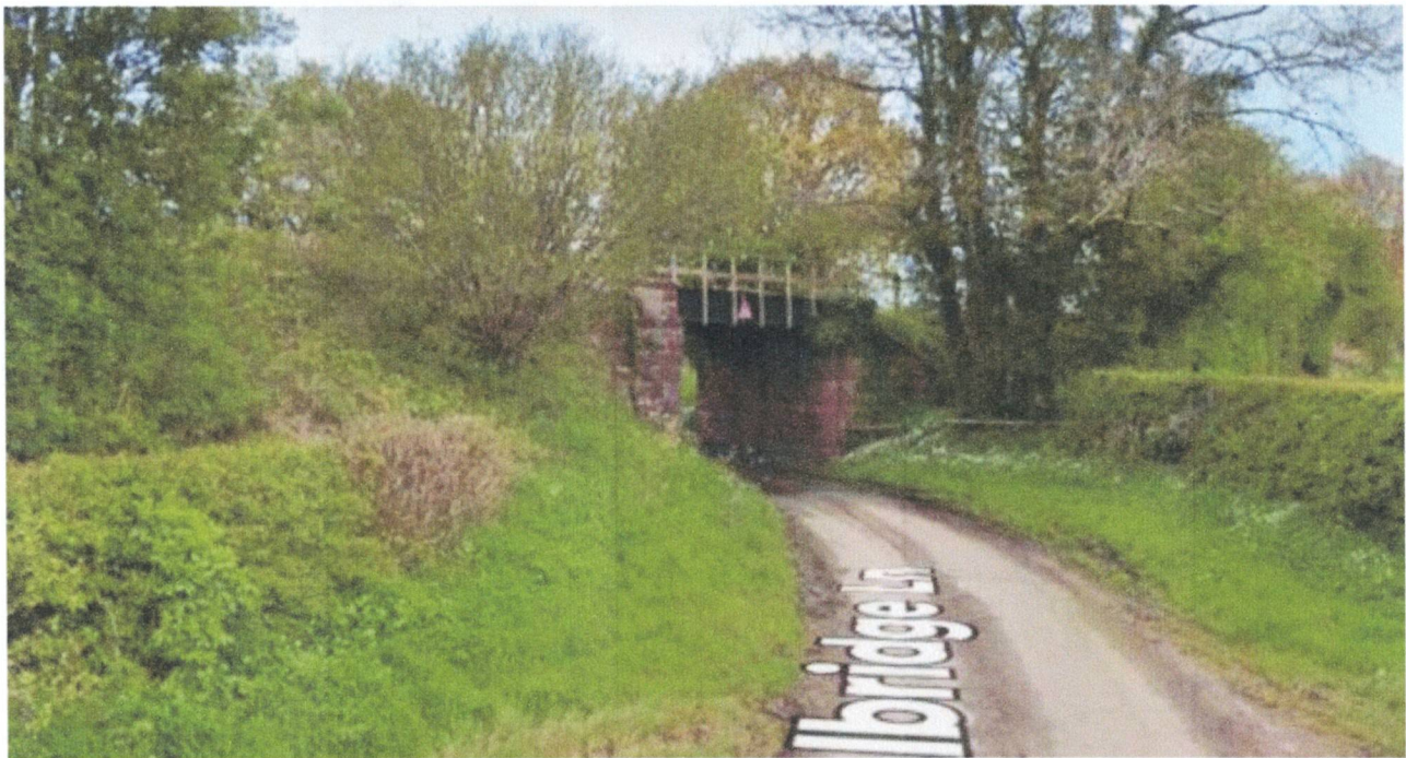
Looking North through the bridge spanning Albridge Lane. [Google Streetview, April 2024]
