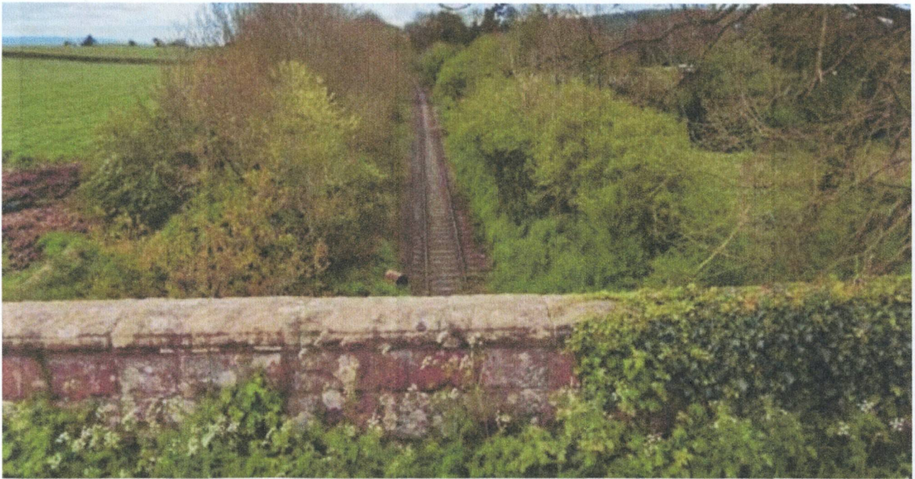
Looking South-southwest from Church Lane Bridge. [Google Streetview, April 2024]
